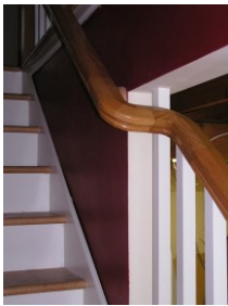
Continuous handrail
