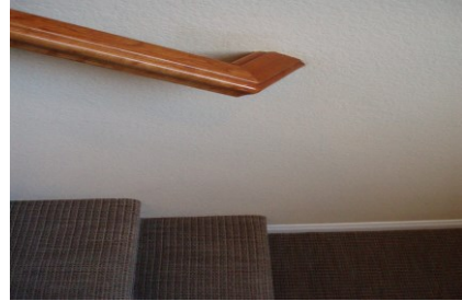
Handrail ends shall be returned toward a wall, guard walking surface continuous to itself, or terminate to a post.
