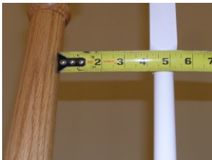
Guards measured at widest opening
