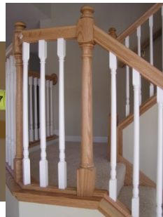
Guards measured at widest opening
