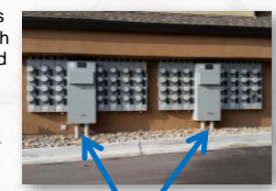
Single Service (both sets of service wires originate from same location)
