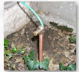
This 1/2" ground rod is listed as an electrode
