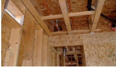
R502.7 except. 2. In Seismic Design Categories D0, D1 and D2, lateral restraint shall be provided at each intermediate support.
