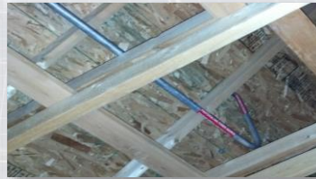
Install by Intermountain Wind and Solar
