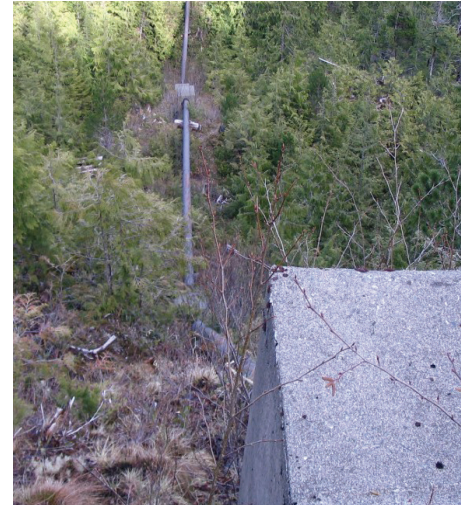
Steep Penstock Drop
