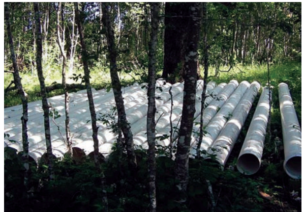
PVC Pipe Ready for Joining and Burying
