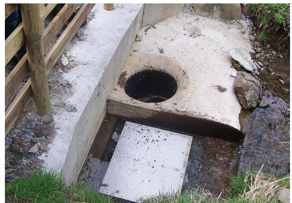
Forebay and Submerged Penstock Entry
