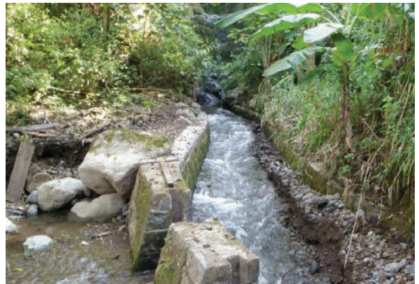
Below Settling Basin After Cleanout - USDA Photo
