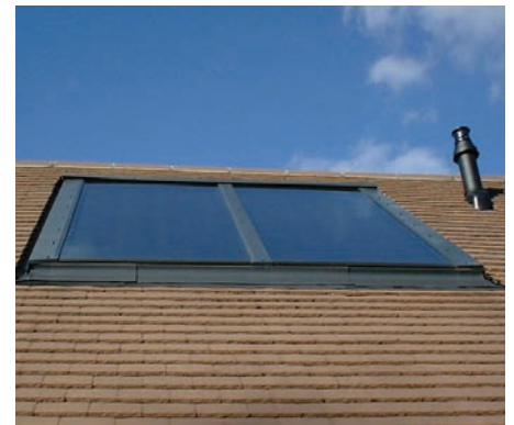
Integrated Heated Air System
