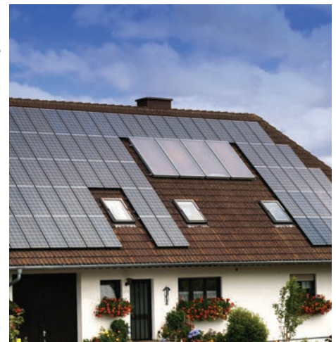
Solar Hot Water Collectors (Middle) Mounted Among Solar Electric Modules
