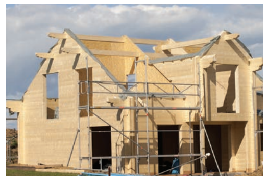
Passive Solar House Under Construction
