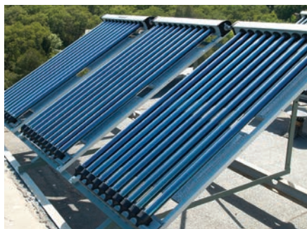
Evacuated Tube Collector
