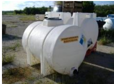
Sodium Hypochlorite: a corrosive. MAQ 500 gallons
