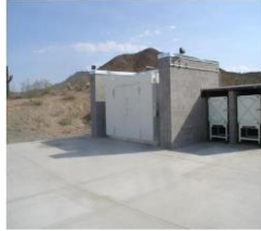
Type 2 Magazine housing 900 lbs of Division 1.1 mass detonation explosives with bullet resistant CMU wall around. Alt. methods and materials used since no panic hardware and no sprinklers allowed per BATFE which takes precedence over IFC/IBC.
