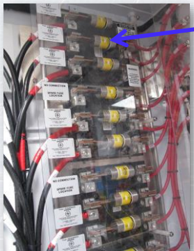
Re-combiner within a central inverter
