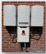
SolarEdge® SE66.6kUS String Inverter
