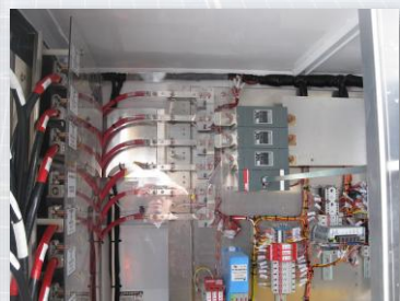
Re-combiner within a central inverter
