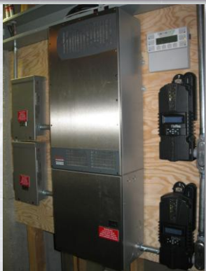
Example of older battery backup PV system (does NOT have the UL 9540 listing)
